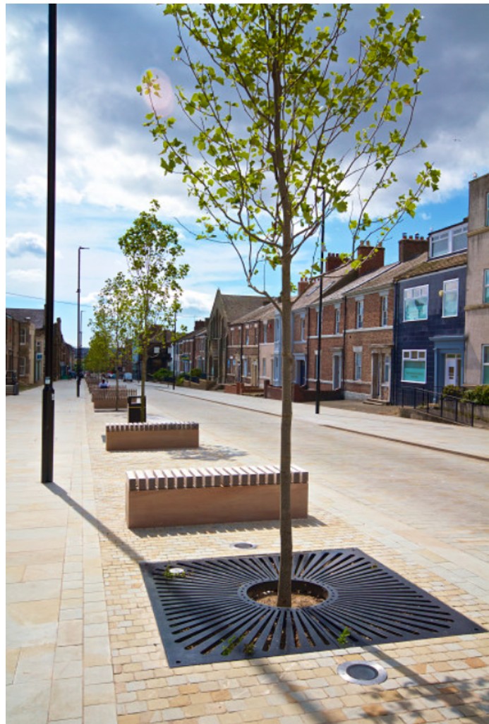
Photo 4.1: Howard Street, North Shields
